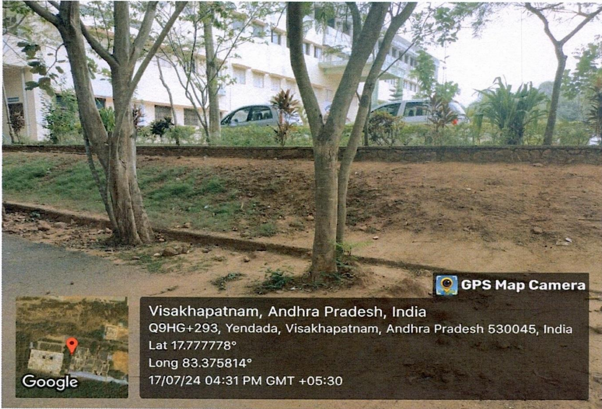
Construction Of Bunds In Block C
