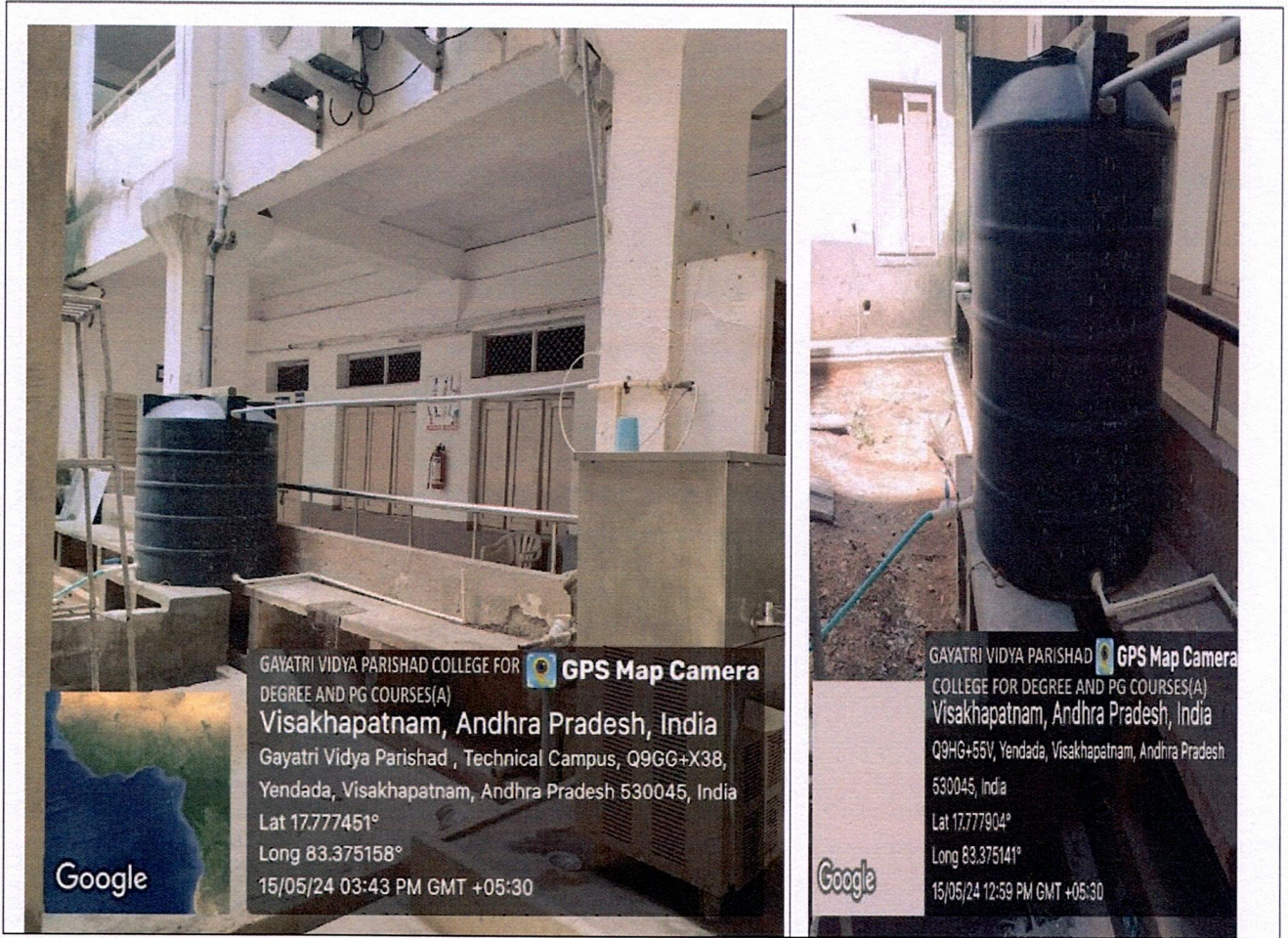
Use of RO Reject Water for cleaning and watering plants in Block C
