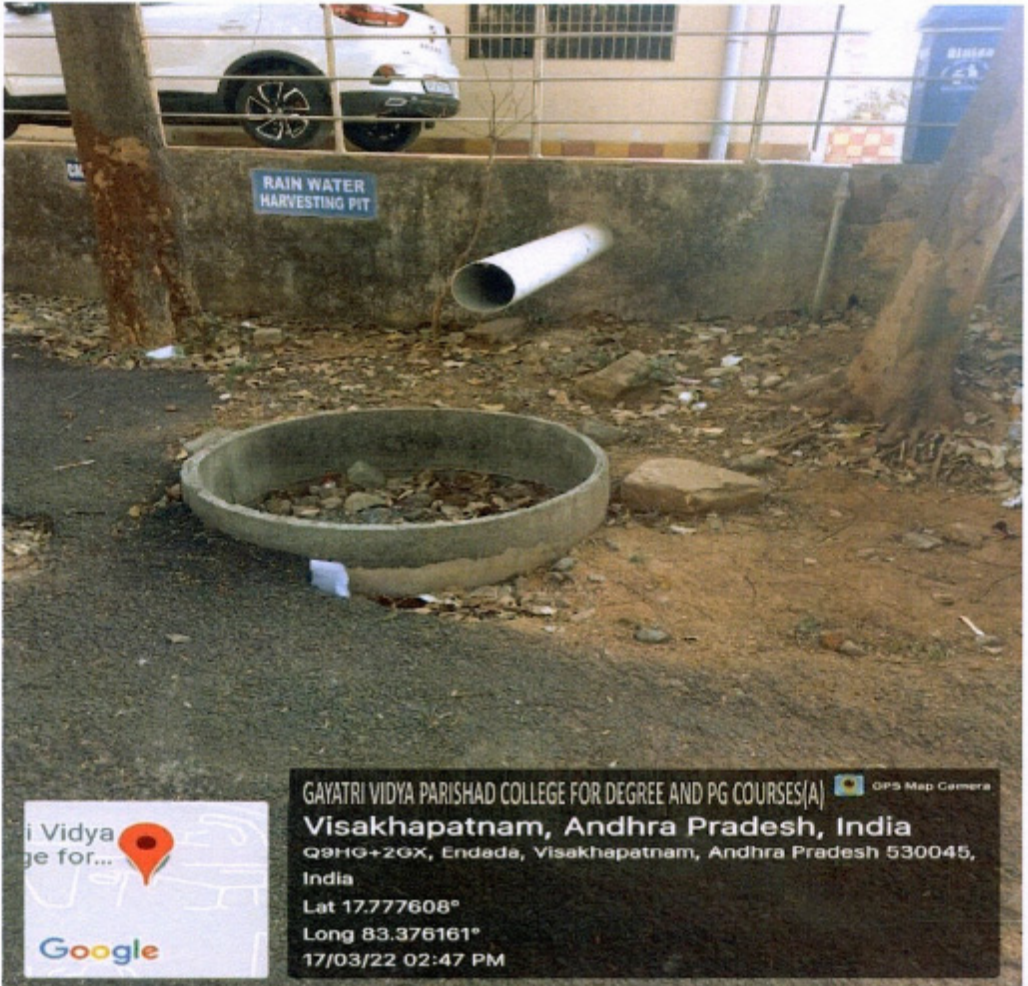
Rain water harvesting pit at Block C Parking area Rushikonda
